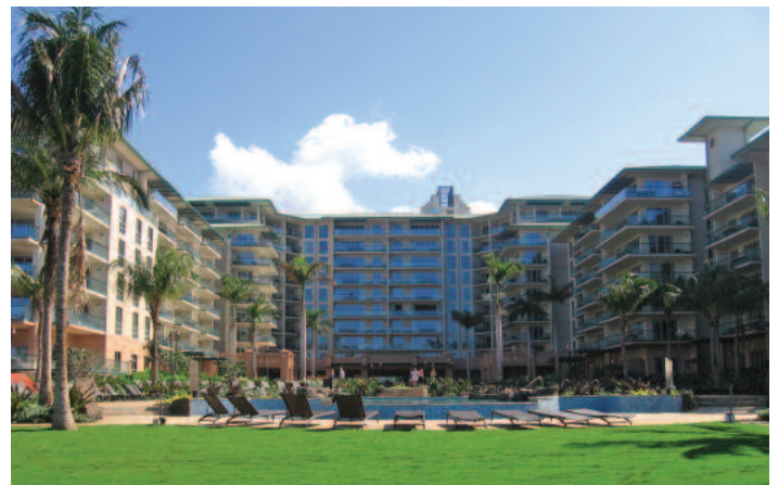
Completed Hokulani building
