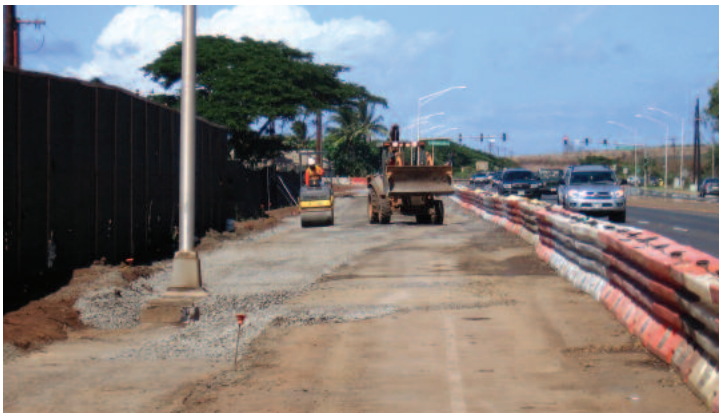
Maui crew widening Honoapiilani Highway for the Honua Kai project
