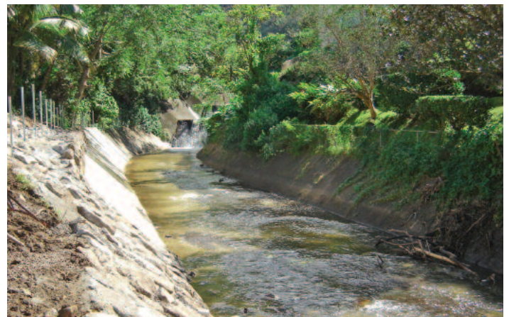
Completed Nuuanu Stream Project
