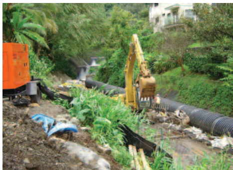
Stream channel diversion system
