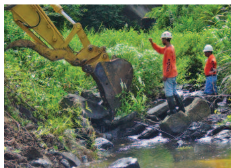
Cheyne Pratt and Flor Mendoza doing initial stream entry work
