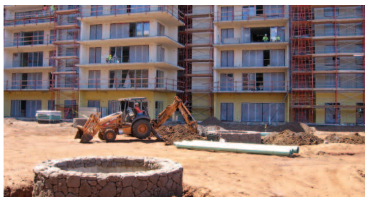
Honua Kai job in progress
