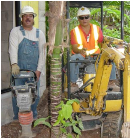
Henry and Gil at Hale Koa Hotel Pantry Renovation
