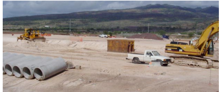
Honolulu Advertiser project with Dick Pacific Construction
