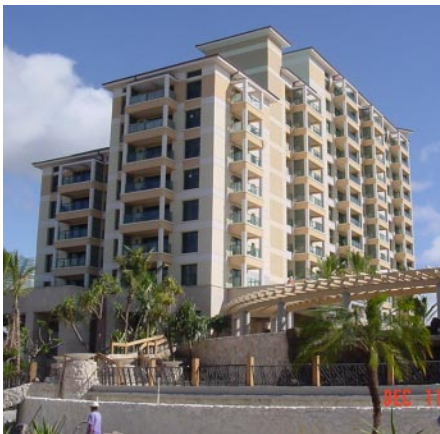
Marriott Ko Olina project with Dick Pacific Construction.
