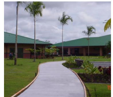
Kamehameha School Phase 2 project with Hawaiian Dredging.
