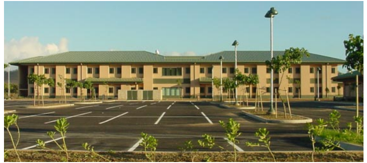
Regional Training Facility at Bellows with Ocean House Builders.
