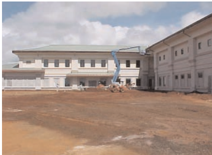
Kauai Police Station with Shioi Construction.
