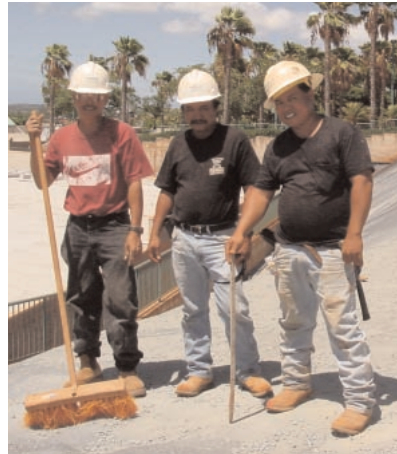
Tom Wong, Flor and "Boy" at the Waikele Retrofit Retaining Walls project.
